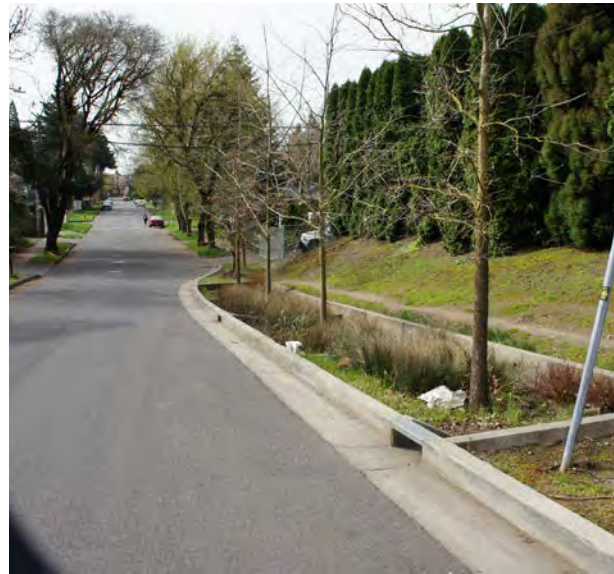
Figure 8: Stormwater curb extensions are a key aspect of the design options. They work to slow and infiltrate stormwater and they are also used to slow traffic down by narrowing the roadway.
