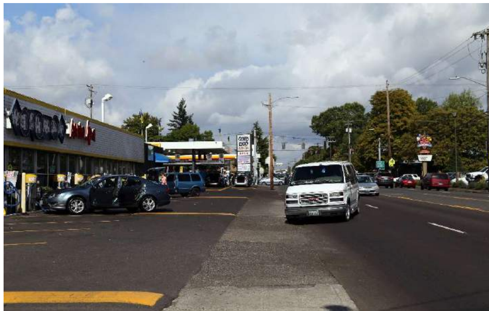
Long curb cut at the Washman Auto Spa. This is anticipated to be remedied at the same time with improvements to the property.
